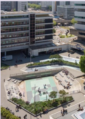
The 'water square' in Rotterdam is a public space that is a playground, while also serving as a water collector in case of heavy rain.
