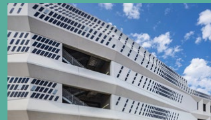
DAZZLE | SAN DIEGO INTERNATIONAL AIRPORT , USA Zero Energy Mediatecture
